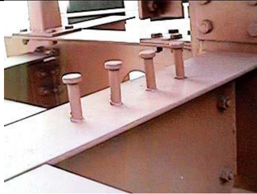
Shear Connectors for Composite Beam
