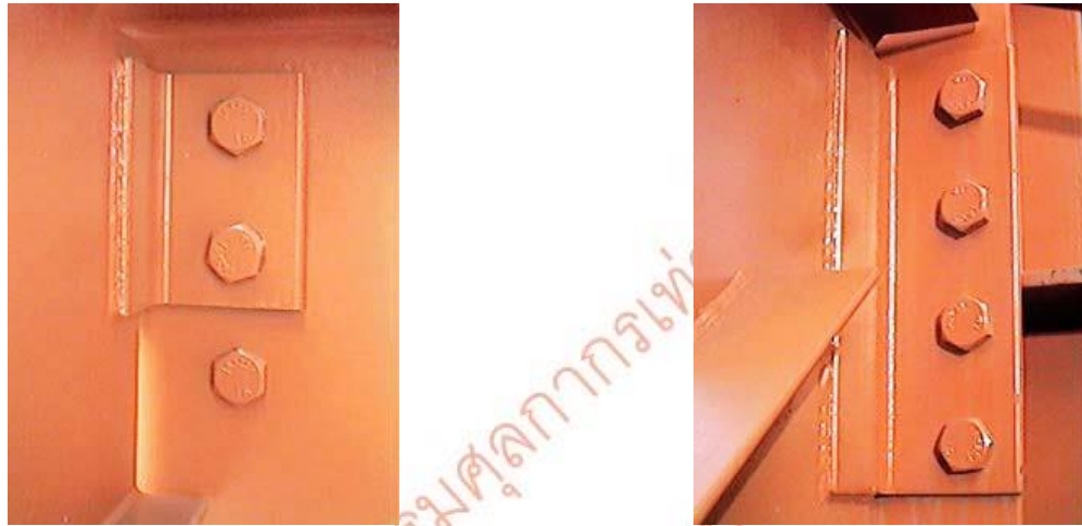
Double Sided Shear Connection
