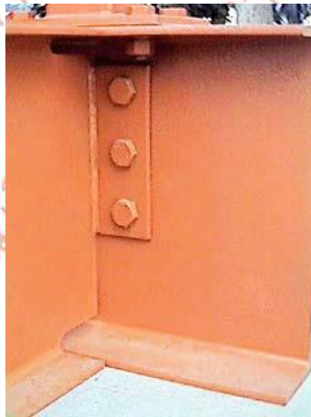
End Plate Shear Connection
