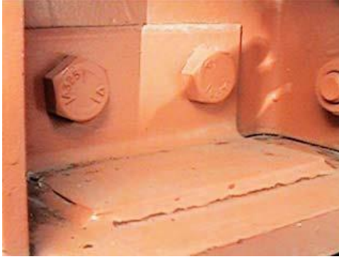
Bolted Top and Seat Shear Connection
