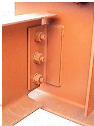
Single Angle Shear Connection
